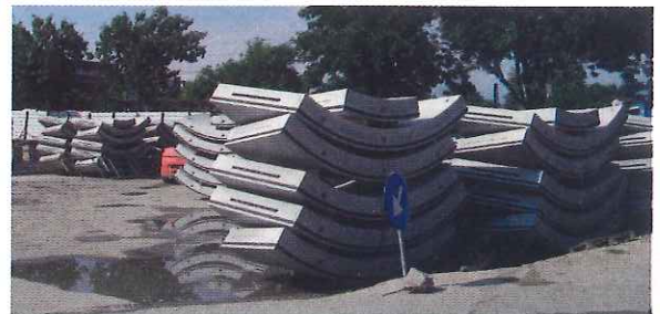
Tunnel lining segments await placement at the Razoare construction site southwest of the city centre.
